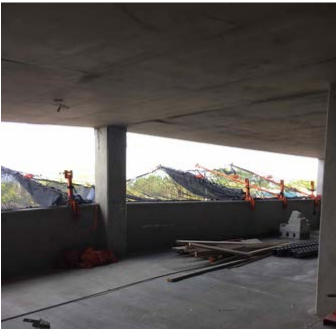
SAFETY NETTING INSTALLED
